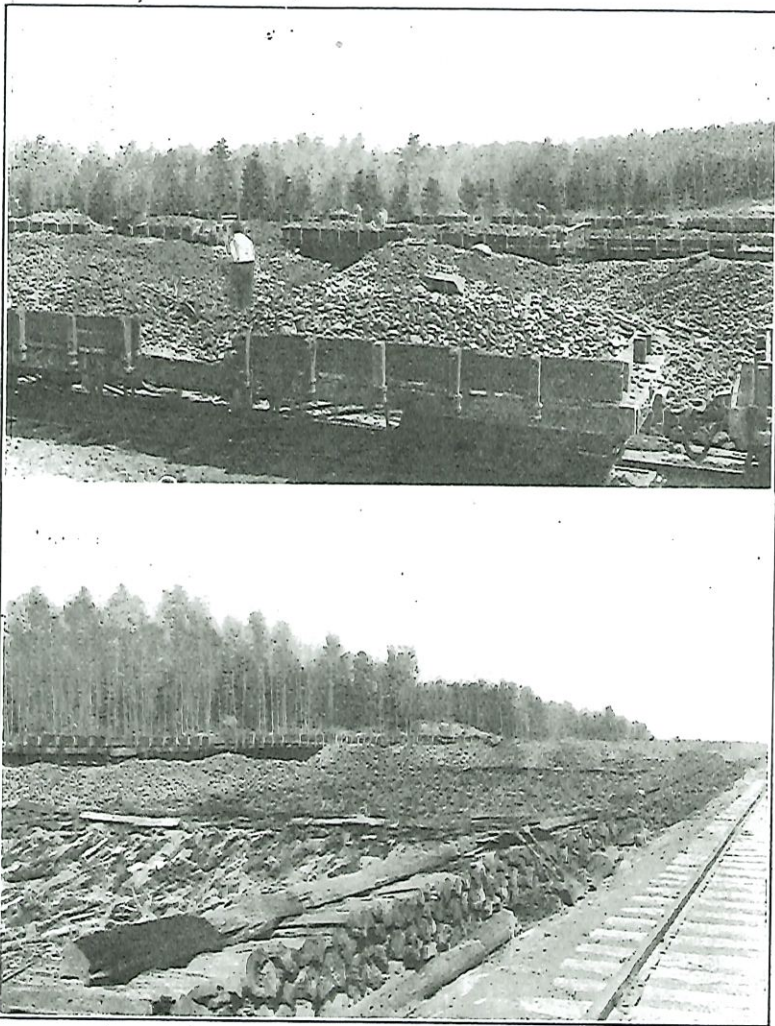
Plate XVI.—Unloading green ore by hand. Plate XVII.—View of roast beds built by hand.
