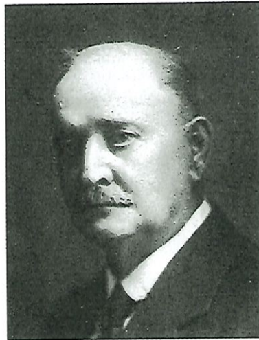
William McVittie c. 1900. He and Frank Cochrane started the Wahnapiatae Power Company in 1902. They fought for and won the right to supply electric power to the city of Sudbury and to Inco and Falconbridge. The generating plant still exists today and is operated by Ontario Hydro. - Inco
