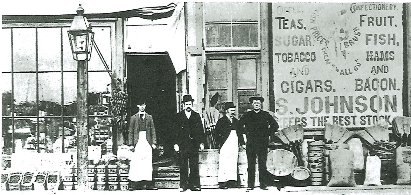
S. Johnson, General Merchant, c. 1894. This store was at the southwest corner of Durham and Cedar streets. – SPL
