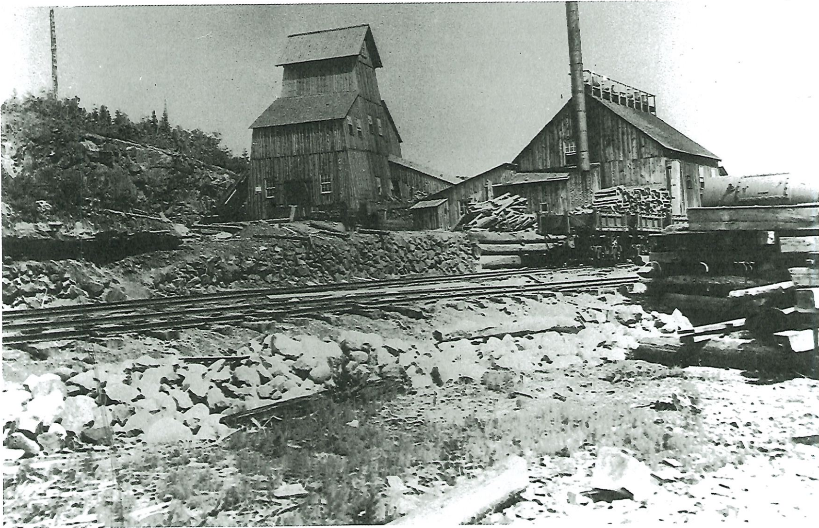
The Copper Cliff Mine boiler house in 1888. The mine shaft is farther left. From the amount of wood piled near the building, it can be assumed the boiler was wood-burning. This view is unusual, as most photos were taken from the other side of the complex. – Inco
