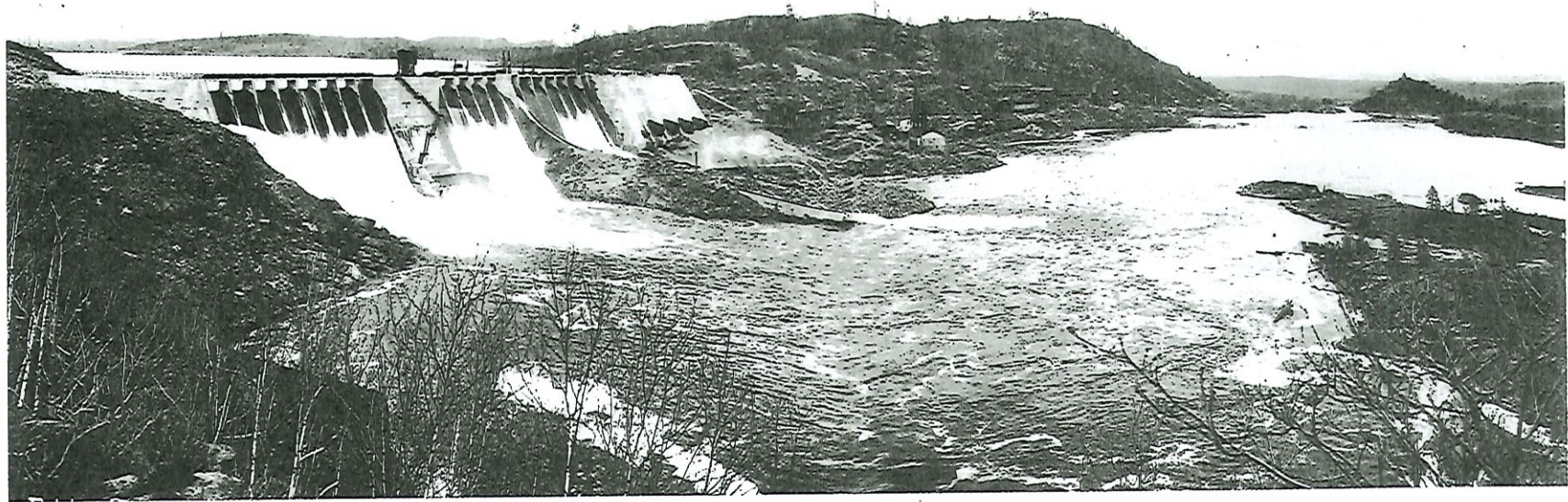
The Big Eddy Dam on the Spanish River west of Sudbury c. 1921. It was was the largest dam in Canada at the time and supplied electricity for Inco at Copper Cliff. The dam is finished but the generating equipment and the buildings to house them have yet to be built. On the far side of the dam are the flues — the four black pipes — that will soon supply the water to turn the turbines. — Inco
