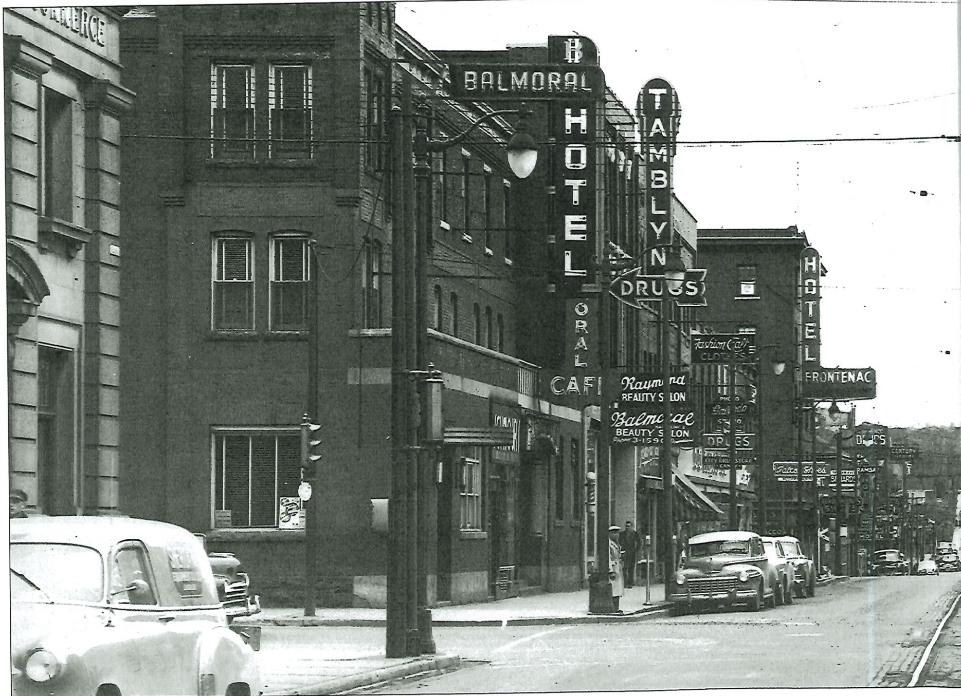
An excellent view of Elm Street in the early 1950s. The Elm Street hill is in the background to the east. The Balmoral Hotel would be demolished in 1957. – D. Farmer
