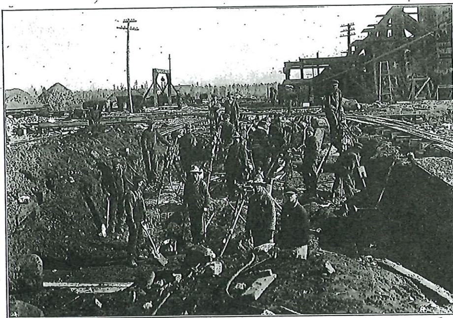
Fig. 66—Commencement of No. 3 shaft, 5 compartments, Creighton mine, 1915.
