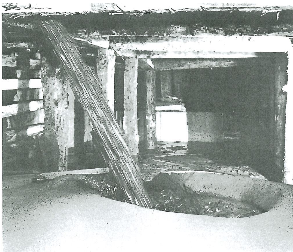
FIGURE 9. Water-borne sand fill flowing into square-set stope.
