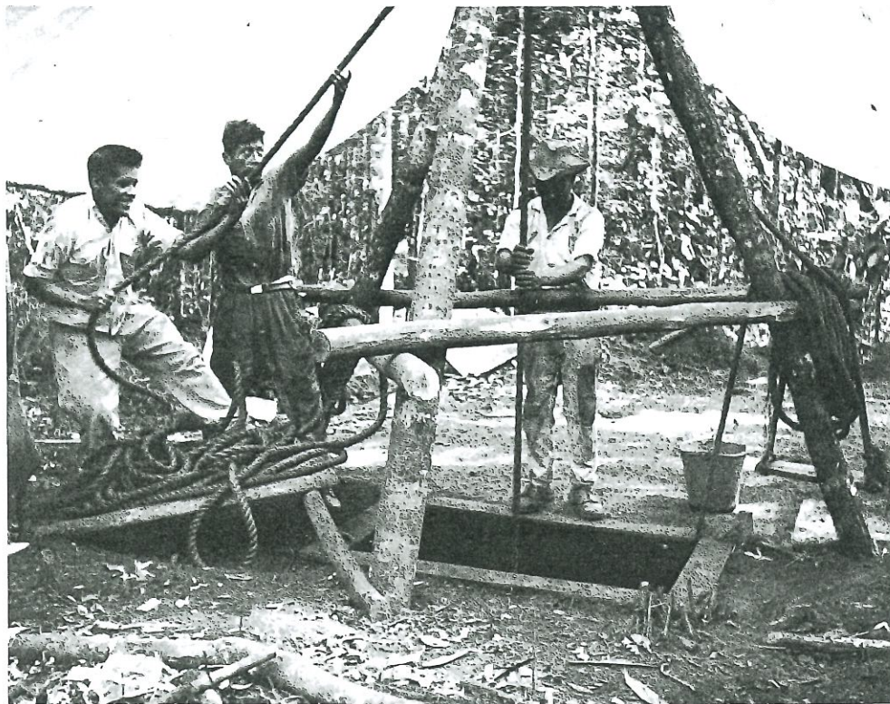
FIGURE 6. Test pit on nickeliferous-laterite deposit, Guatemala.
