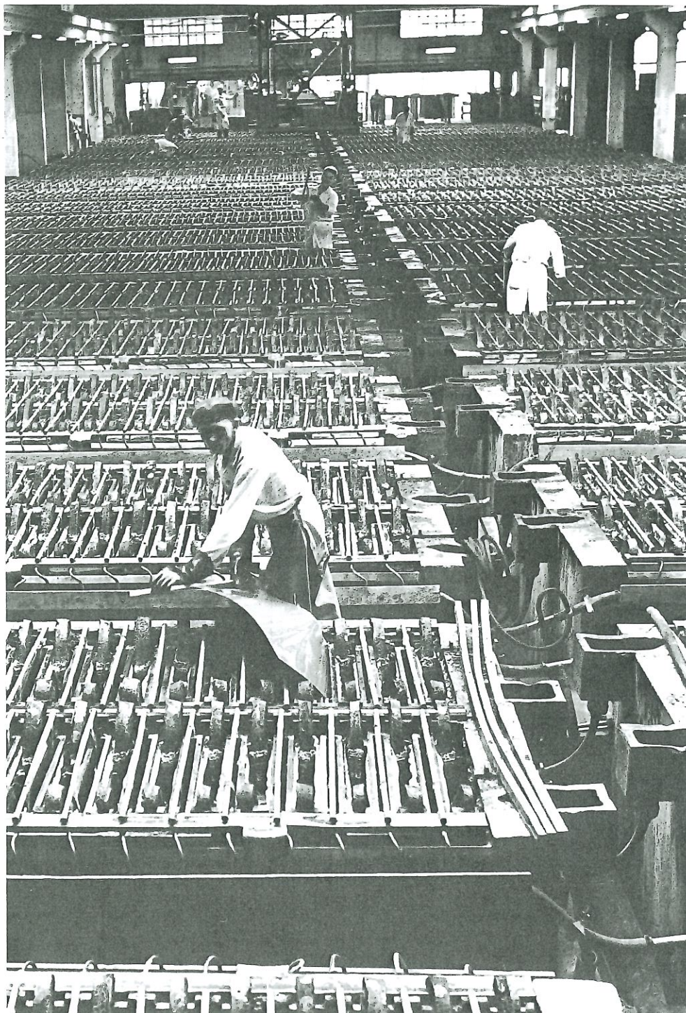
FIGURE 23. Electrolytic nickel refining, Kristiansand refinery.
