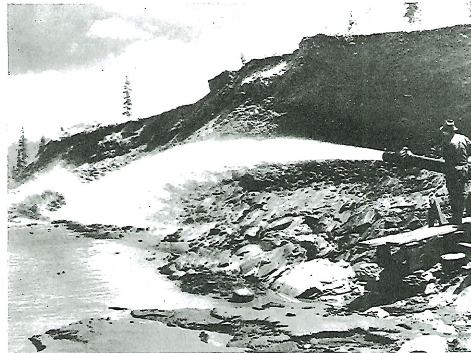
Hydraulic monitor sluicing gold-bearing gravel
