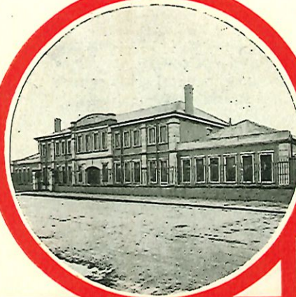
REFINERY Acton, England
