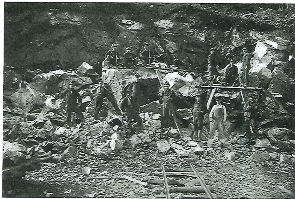
LEVACK MINE. BREAKING LARGE BLOCKS OF ORE IN AN OPEN CAST.
