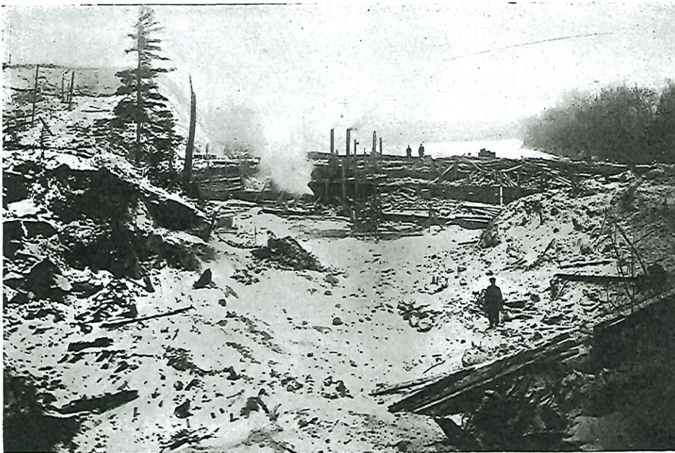
CONSTRUCTION OF NAIRN FALLS PLANT.—SPRING, 1915. SHOWING FIRST COFFER DAM LOOKING UP-STREAM OF SPANISH RIVER.
