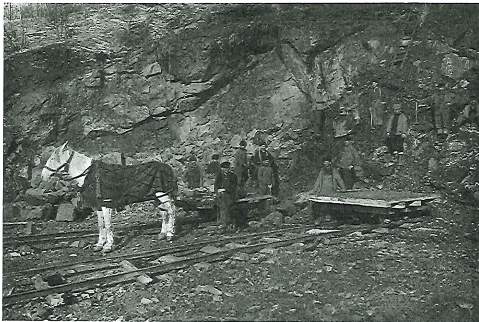
LEVACK MINE. BREAKING SURFACE ORE.
