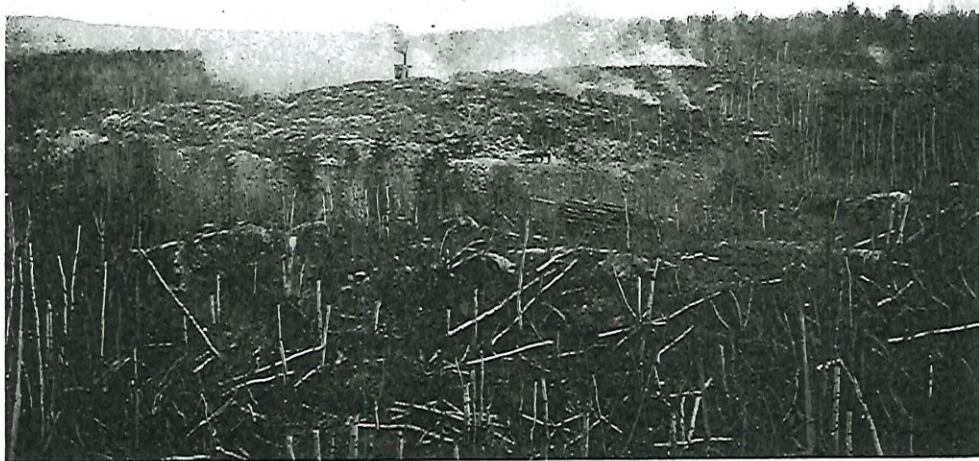
CONISTON SMELTER SITE BEING CLEARED. SEPTEMBER, 1911.
