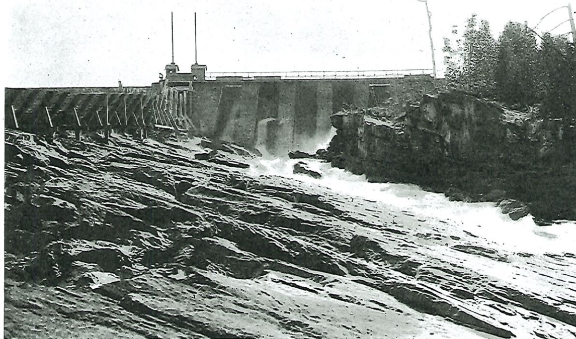
WABAGESHIK POWER PLANT. MAIN DAM AND LOG CHUTE.
