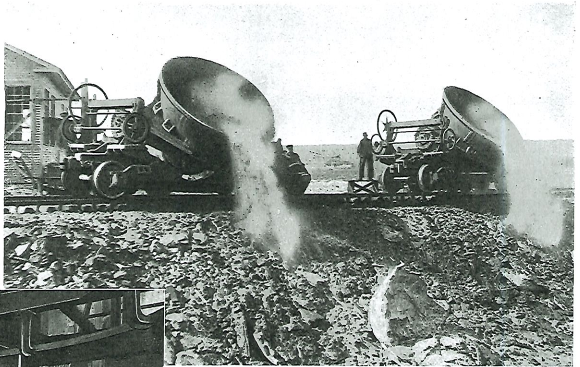
CONISTON PLANT. DUMPING SLAG CARS.
