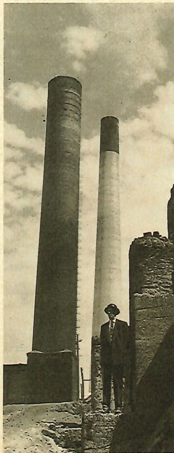
New 400-foot Coniston smelter stack.
