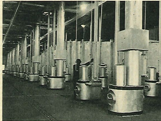
New dust collection cottrels indicated modernization.
