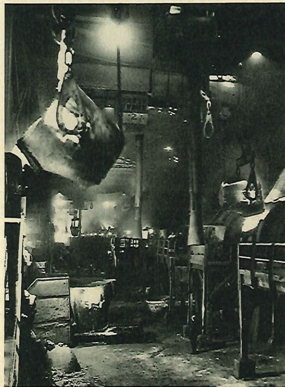
Smelter converter aisle during peak production period.
