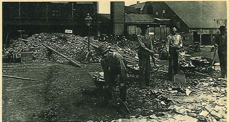
Breaking and stockpiling matte in smelter yard.
