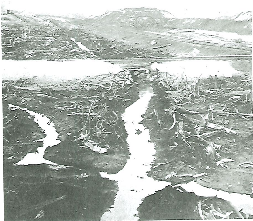
Figure 2.2: Copper Cliff Roast Yard No. 2, c. 1904 ran in a northeasterly direction from the present School Street to halfway down Cobalt Street, although it was popularly thought to have been located in Nickel Park. The yard's dimensions were 1,000 feet by 125 feet, and it operated from 1899-1903. Raw ore was roasted over wood fires to remove sulphur from the ore, a process which could consume one to seven months, depending upon the amount of ore heaped in the yard. Subsequently, the roasted ore was transported to a smelter. (Laroche and Sirois 1979)
