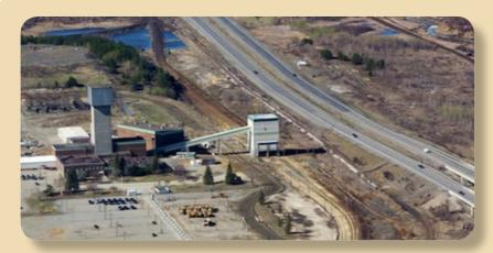
**View 2:** An aerial view of the inactive Copper Cliff (South) Mine, showing the headframe on the left. Regional Road 55 is in the upper right. When the headframe was active, ore was raised from the mine and moved by an inclined conveyor to ore bins in the white building above railway tracks, where it was loaded in rail cars for shipment to the nearby mill. *Photo courtesy of the Ontario Geological Survey.*
