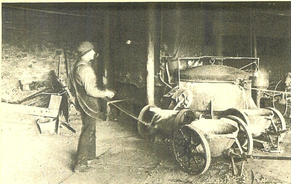
Primitive, but effective first smelting at Copper Cliff.
