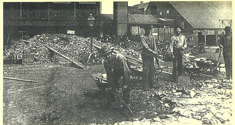
Breaking and stockpiling matte in smelter yard.
