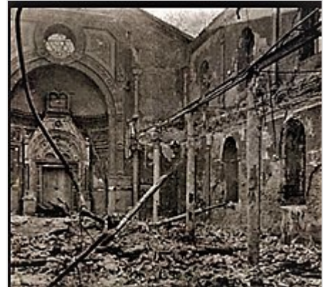
Synagogue in Bucharest after it was set on fire during a pogrom, January 1941
