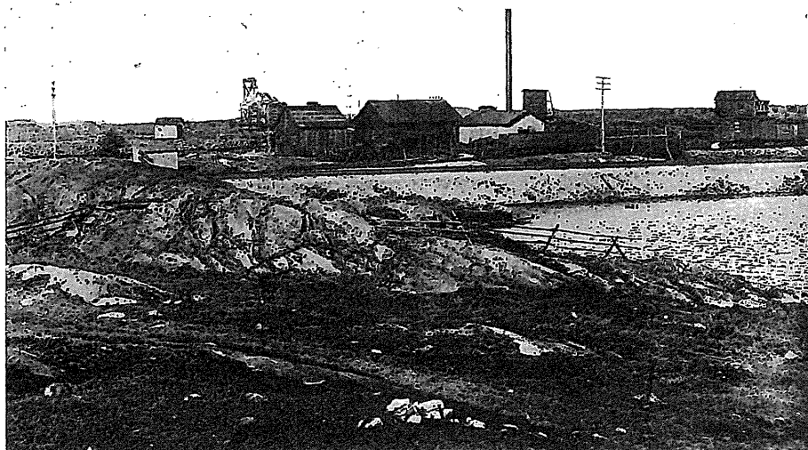
Fig. 53—Murray mine, Sudbury area, Ontario, September 2nd, 1916. A modern plant and smelter are being erected at the Murray mine by the British America Nickel Corporation.
