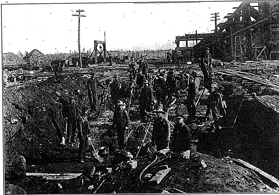
Fig. 66—Commencement of No. 3 shaft, 5 compartments, Creighton mine, 1915.
