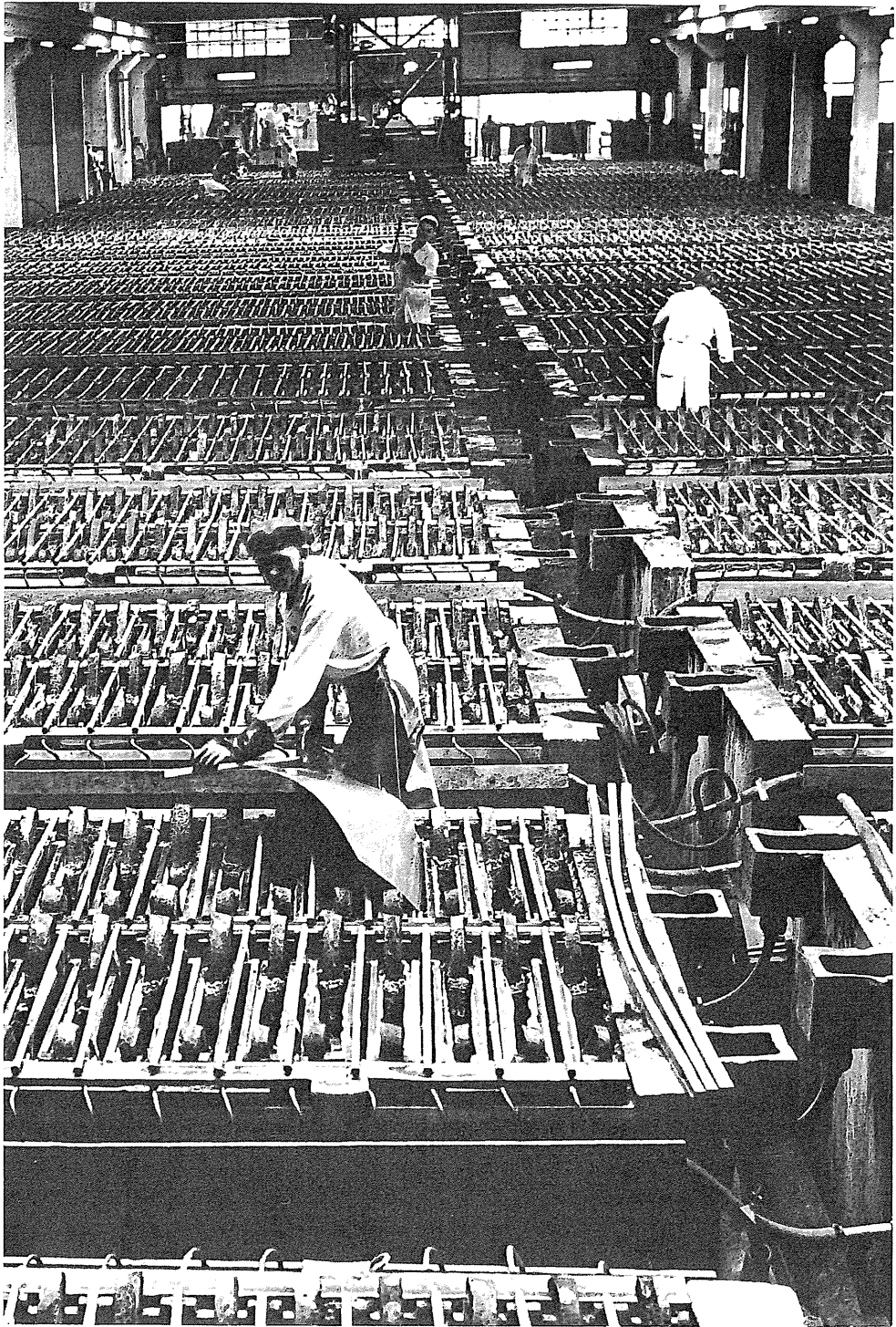
FIGURE 23. Electrolytic nickel refining, Kristiansand refinery.
