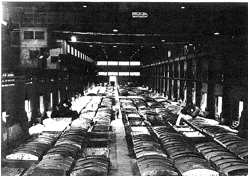
FIGURE 20. Matte casting and cooling, Copper Cliff smelter.
