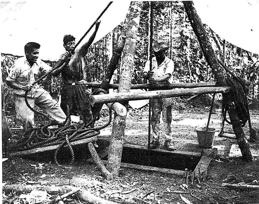
FIGURE 6. Test pit on nickeliferous-laterite deposit, Guatemala.
