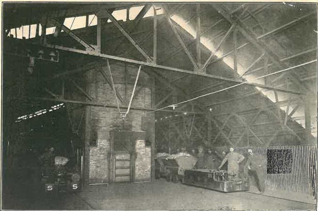
Charging floor, blast furnace plant, Canadian Copper Co., Copper Cliff, Ont.
