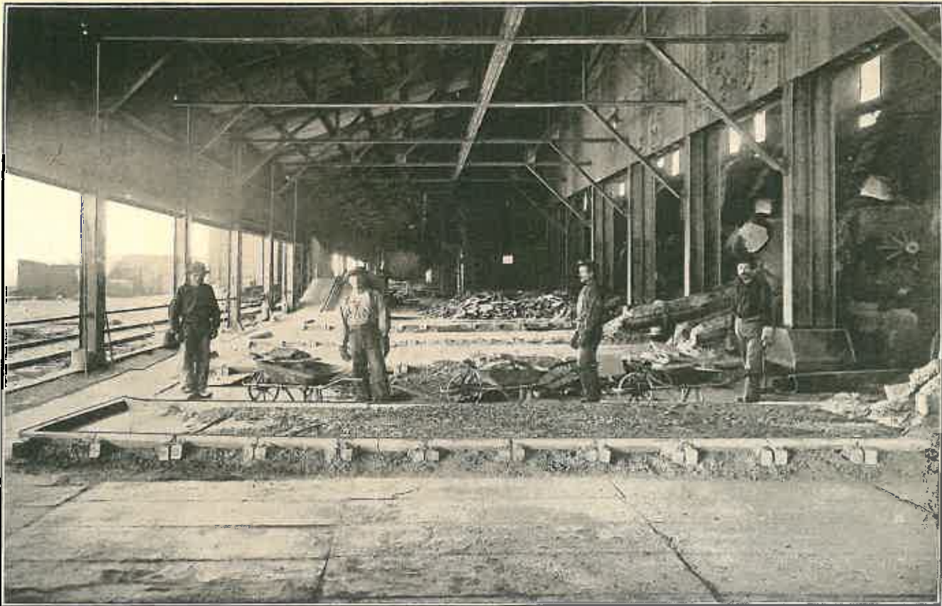
Interior of matte shed, Canadian Copper Co., Copper Cliff, Ont.
