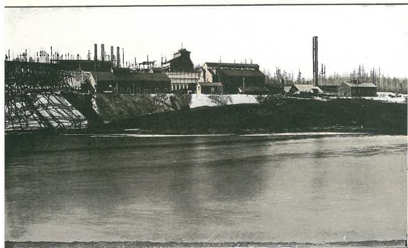
Ladysmith smelter, Tyee Copper Co., Ladysmith, B.C.
