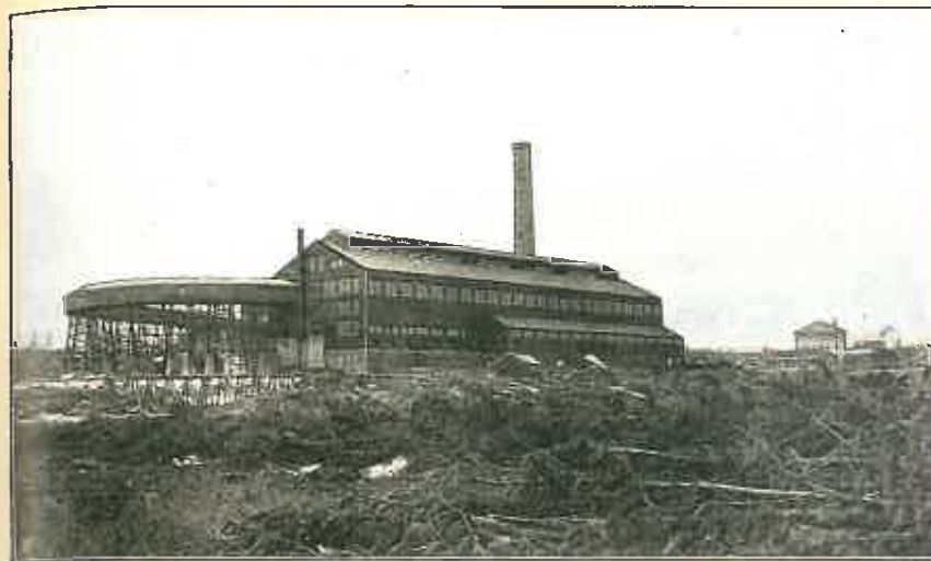
A. General view of the completed plant at Coniston. Note the curved line of trestles carrying the tracks that run under the ore bins and on the charging floor level.
