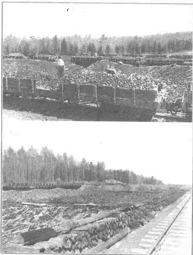
Plate XVI.—Unloading green ore by hand. Plate XVII.—View of roast beds built by hand.
