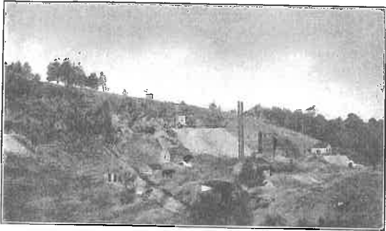
Fig. 2—Mill and other mine buildings, Renfrew Molybdenum Mines, Ltd., lots 8 and 9, con. XI, Brougham tp., Renfrew county, Ontario.
