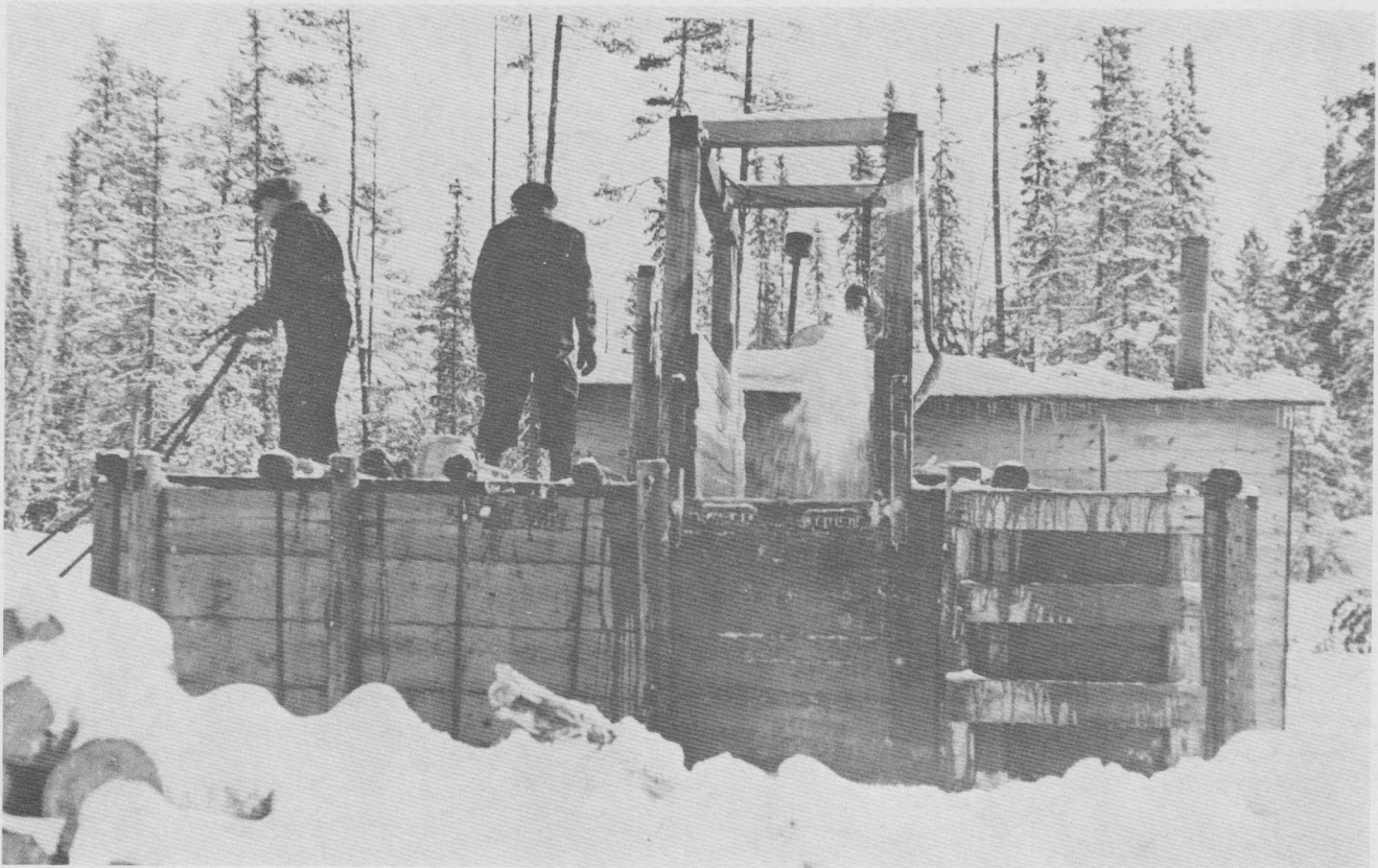
36. Filling the tank sled to ice the hauling roads.
