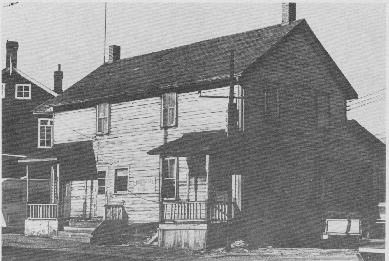
204. C.P.R. double house, Frood Road, built 1894-5.
