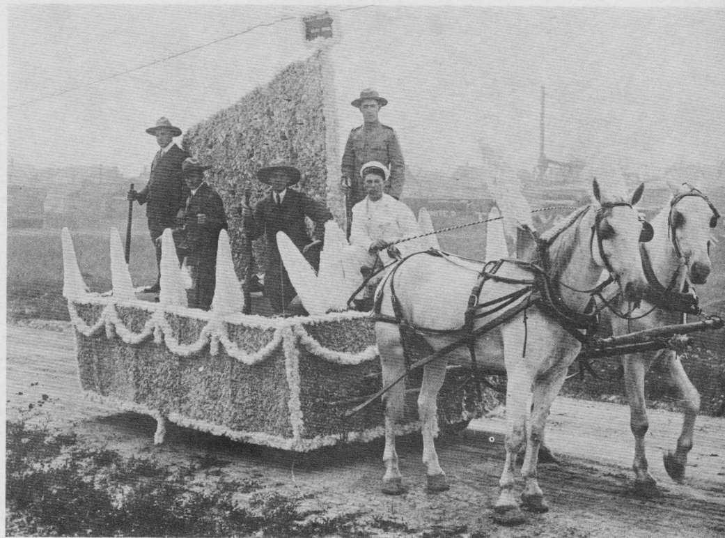
152. Wilson & Greenwood's entry, July 1st parade 1914. Evans' lumber mill in background.
