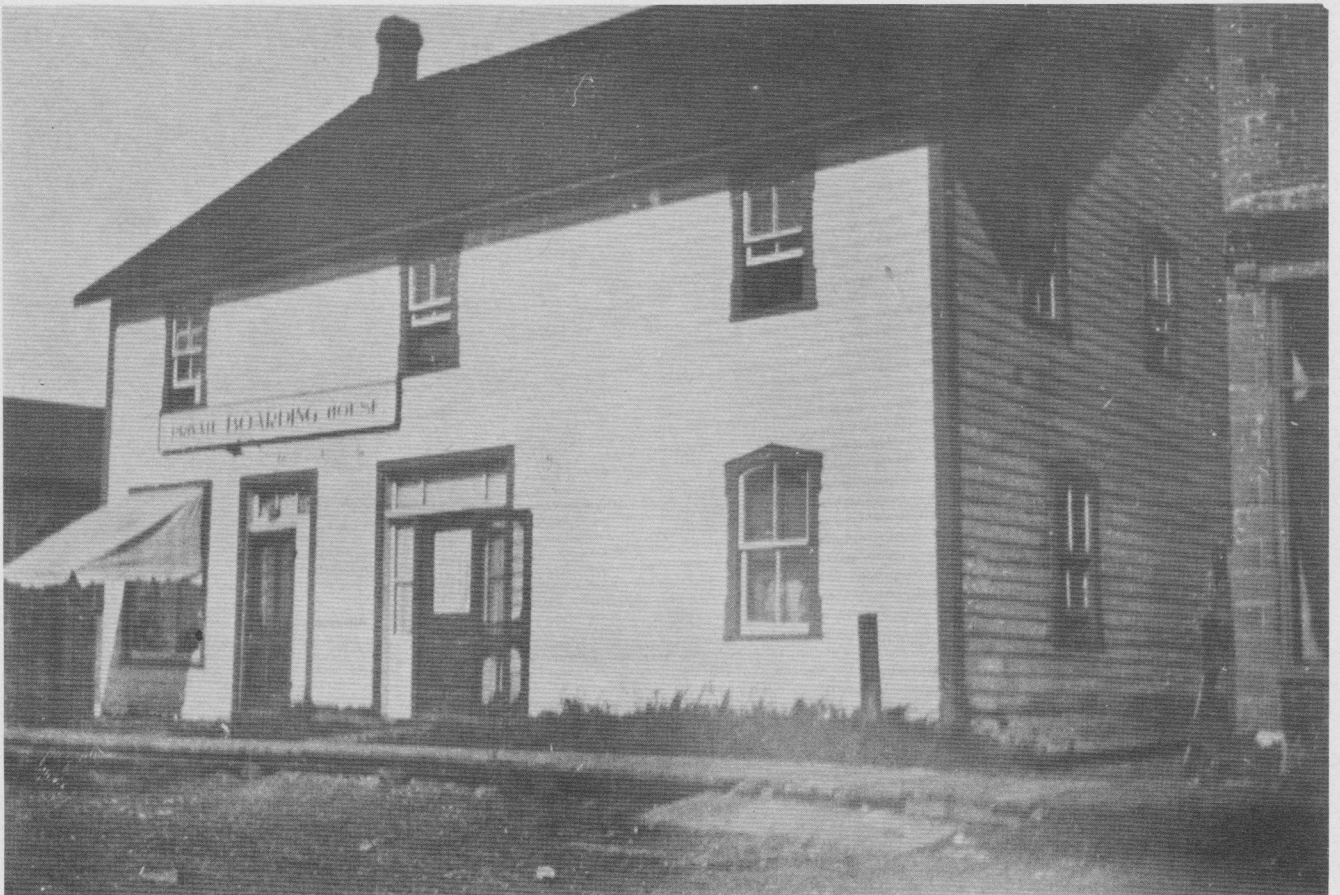
118. Peloquin boarding house, Elgin Street, 1906. At right Moses Block under construction.
