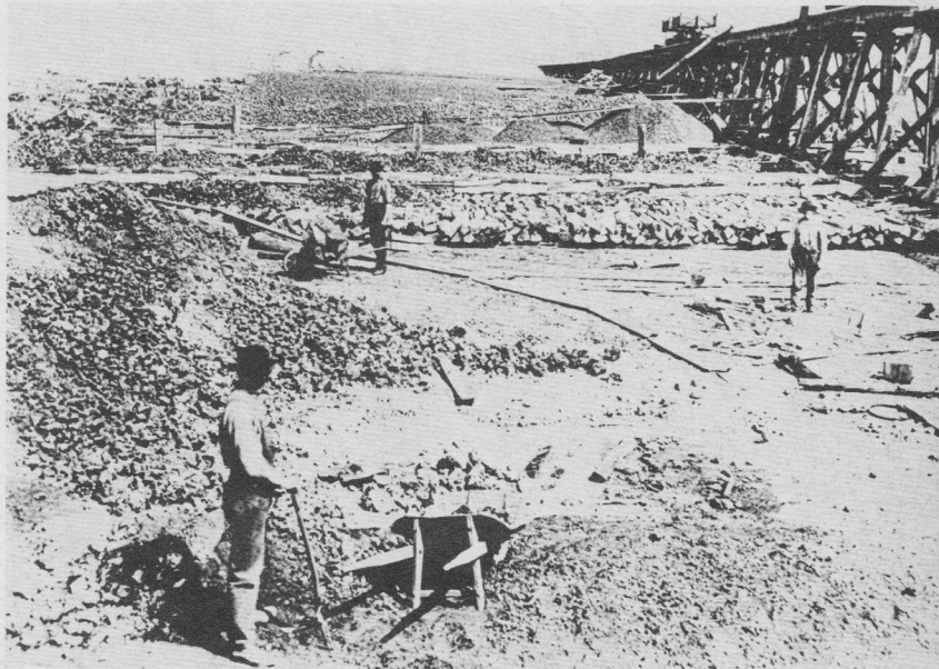
56. Unloading green ore from jimmy cars, Copper Cliff roast bed, 1889-90.
