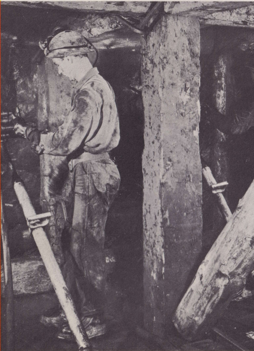
Drilling operations in a square-set stope.
