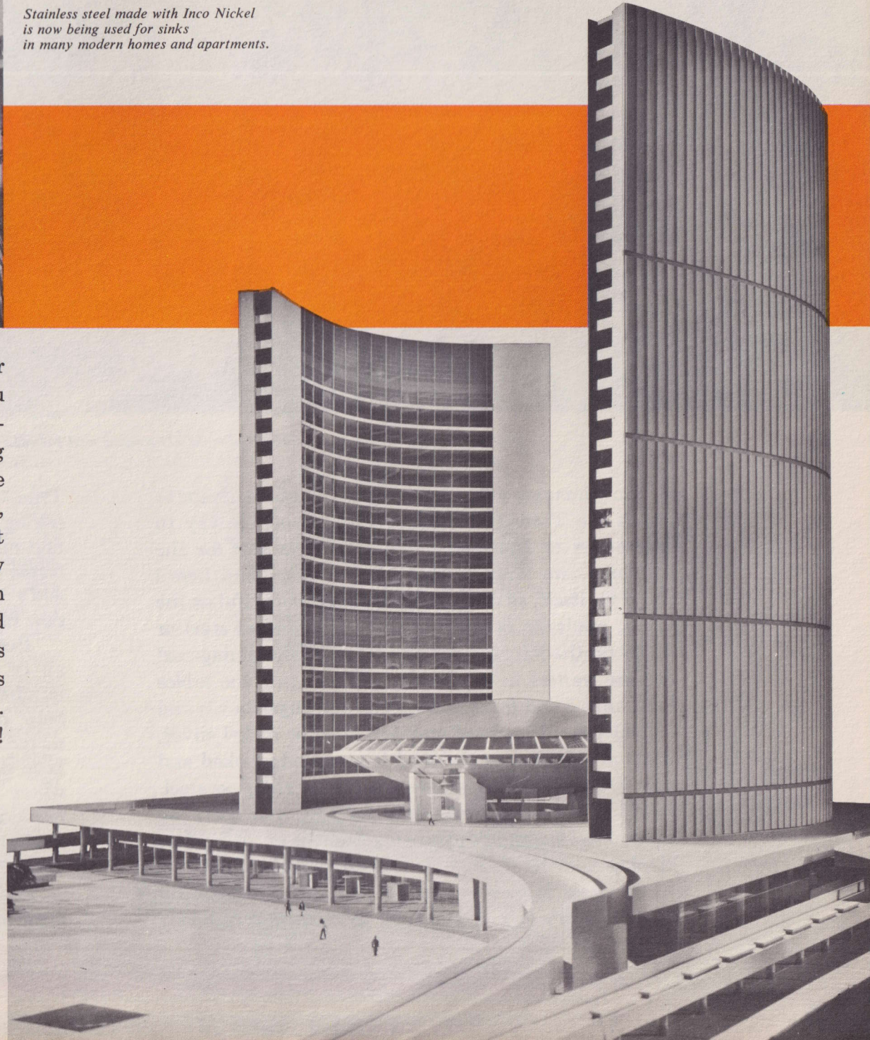
Nickel stainless steel is used in the window frames and doors of Toronto's modern new City Hall.
